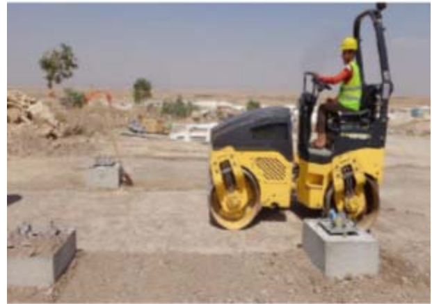
Filling For Foundation
